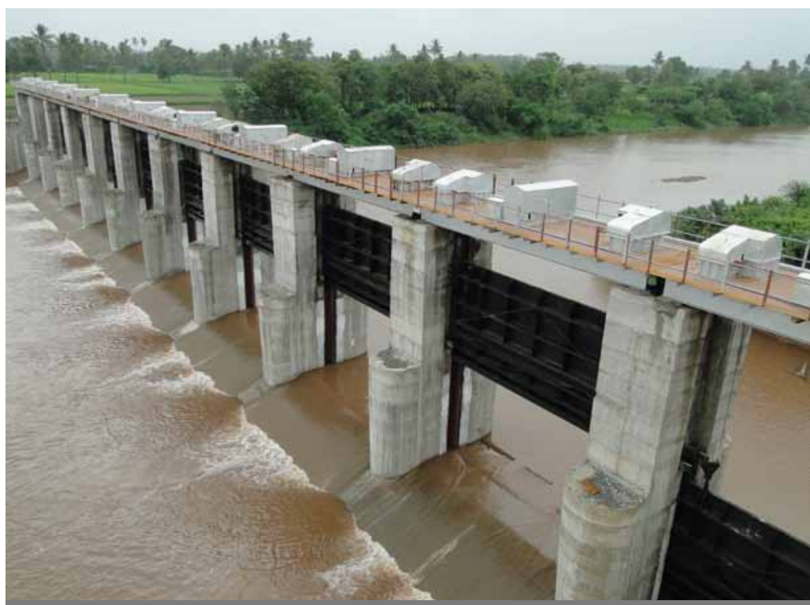
Bhakeshwar Dam near Kodinar (Gujarat) got completed in 2013 at a total cost of over ₹12 crores (40% shared by the Company and 60 % by Gujarat govt.). The dam has a storage capacity of 1.41 million cubic meters providing water security and irrigation benefits for second and third crops in about 1,167 hectare area consisting of 1,150 wells within 8 coastal villages. Additional recharge of water through the dam will also prevent salinity ingress in coastal aquifers thus benefitting these villages.
