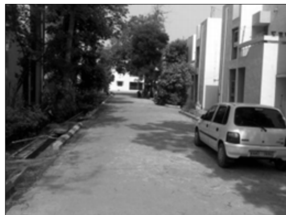
Figure 3. Absence of thermal cracks
