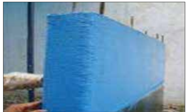
Wrapping with carbon fiber
