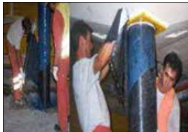
Wrapping with carbon fiber
