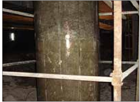
Surface primer applied on the column
