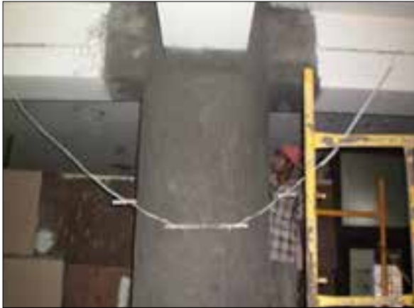
Surface grinding and prepared for fibre wrapping
