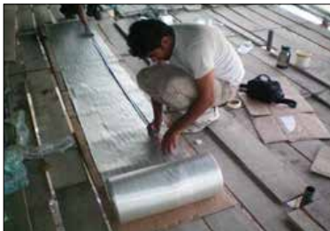
Cutting of fibre sheet
