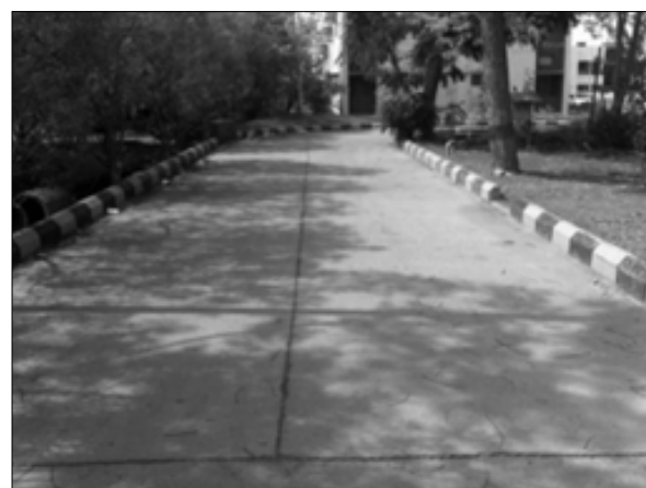
Figure 2. Absence of shrinkage cracks
