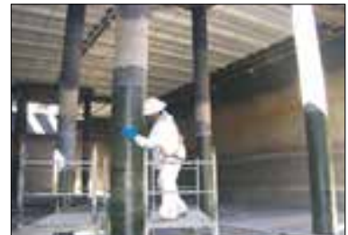
Wrapping with carbon fiber
