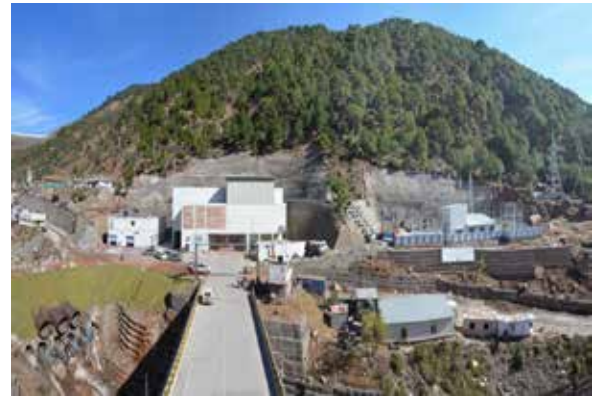
Figure 2. Outer Tunnel View
