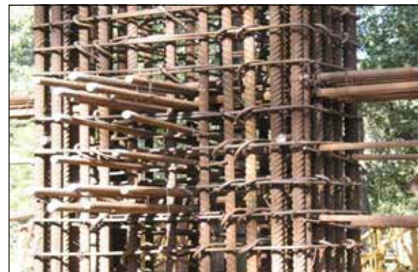
Figure 3: Impurities in Steel Rebars
