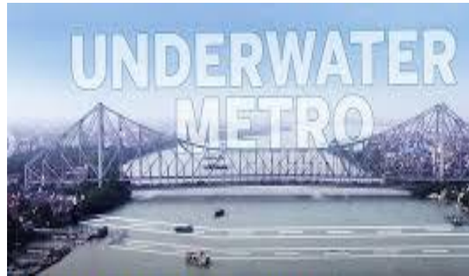
Kolkata's Underwater East West Metro Tunnel
