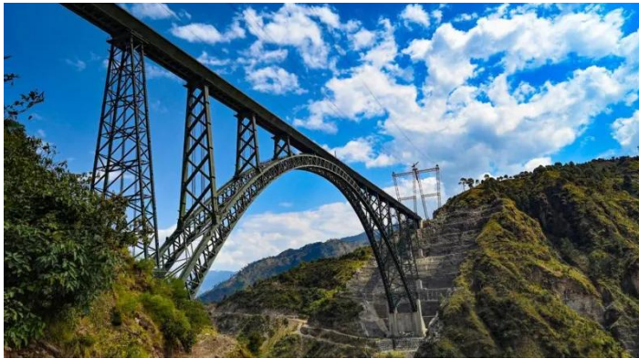
Chenab River Arch Bridge
