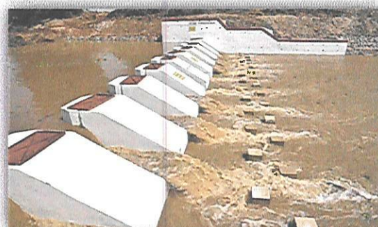
Masonry Check dam on after completion of construction work
