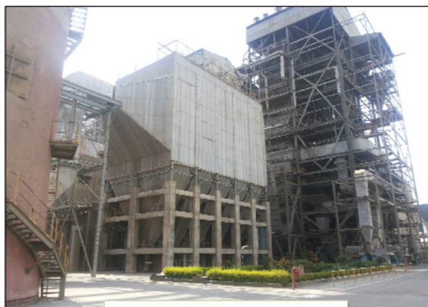
ESP to control Dust emission at source
