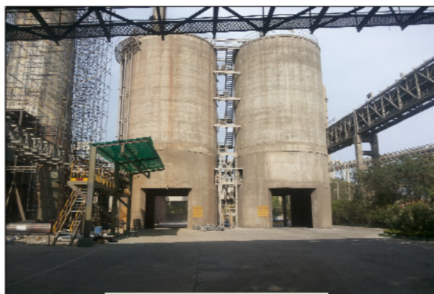
Properly covered Fly ash storage silo
