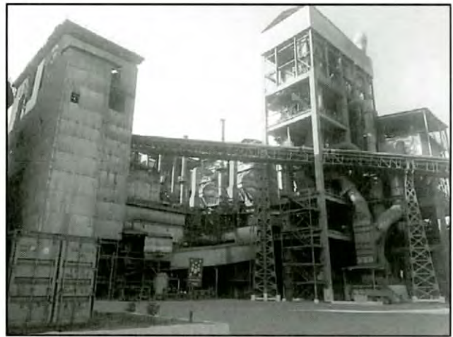
Bag House at Klin Stack
