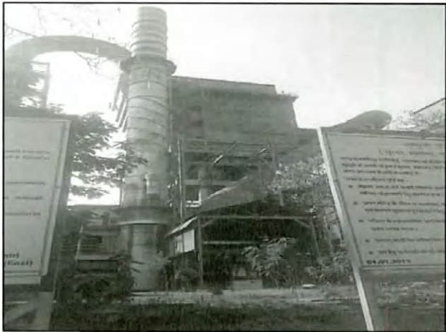
Bag House at Klin Stack
