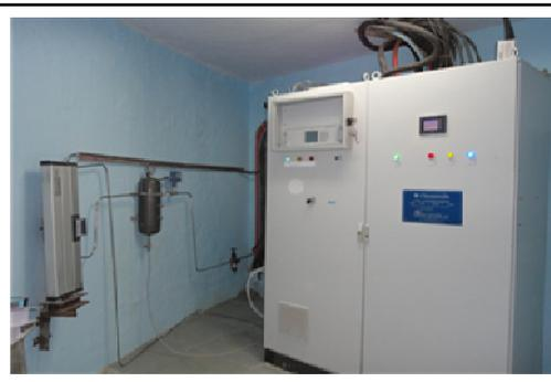
CEMS - The MCS100E IR-Analyzer, SICK MAIHAK GmbH is used for continuous selective measurement of pollutant substances
