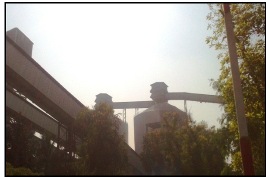
Fig 2 : Covered Conveyors
