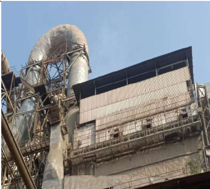
Hybrid filter at Raw Mill
