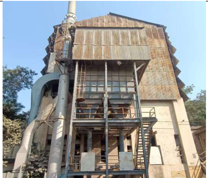
Bag Filter at Crusher Stack
