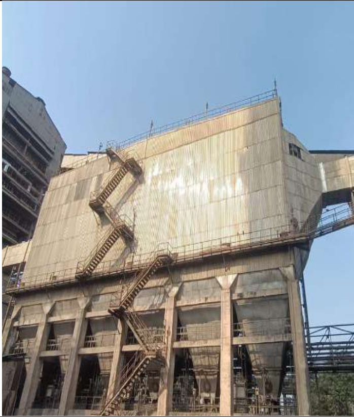
ESP at TPP 15 MW
