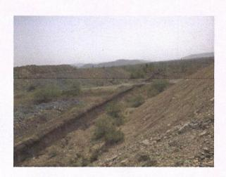
iv. Garland drain (size, gradient and length) shall be constructed for both mine pit and sump capacity should be designed keeping 50% safety margin over and above peak sudden rainfall (based on 50 years data) and maximum discharge in the area adjoining the mine site. Sump capacity should also provide adequate retention period to allow proper settling of silt material. Sedimentation pits should be constructed at the corners of the garland drains and desilted at regular intervals.
