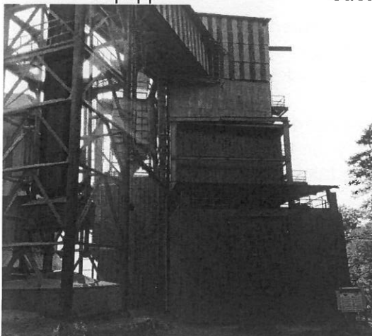
BF installed at material transfer point
