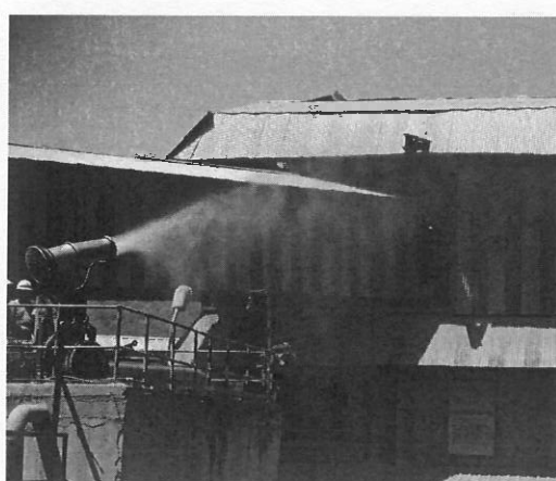
Water fogger system installed at Crusher
