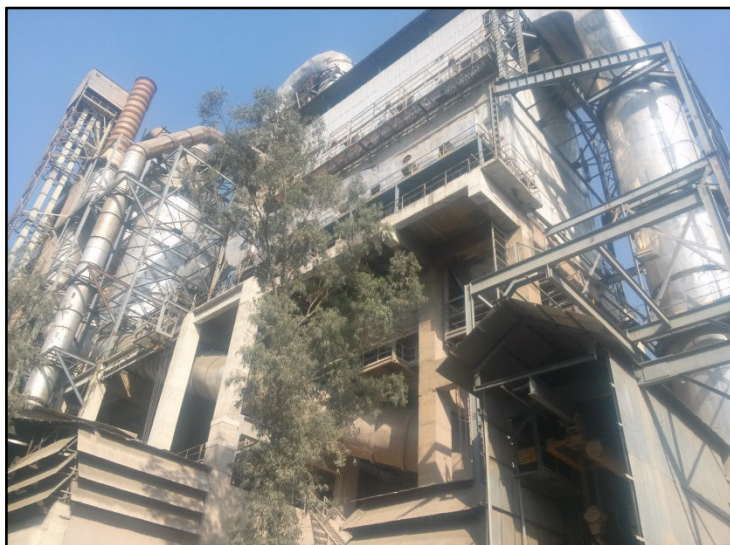
Hybrid Filter at Cement Mill
