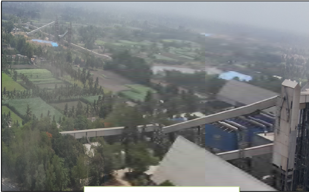
Covered belt conveyor from Coal storage area to Boiler
