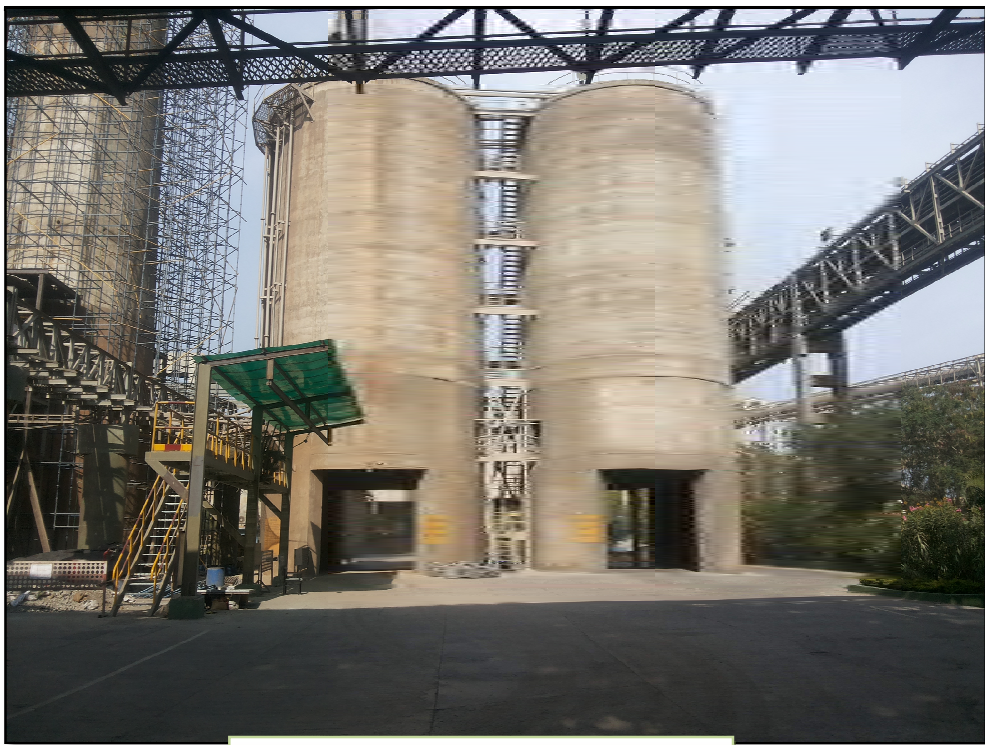
Properly covered Fly ash storage silo
