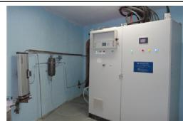
CEMS - The MCS100E IR-Analyzer, SICK MAIHAK GmbH is used for continuous selective measurement of pollutant substances
