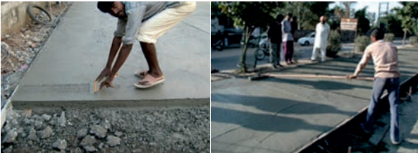
Figure 3: Brooming : Groove cutting
