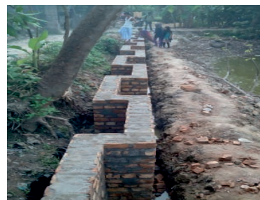
Figure 1: Zig-zag Shape Wall
