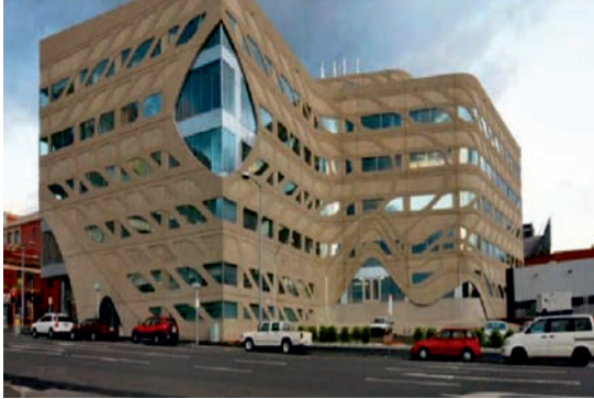
Figure 4: Design, Texture & Colour on concrete precast panels with glass using NOEplast formliners, Hebau deactivators
