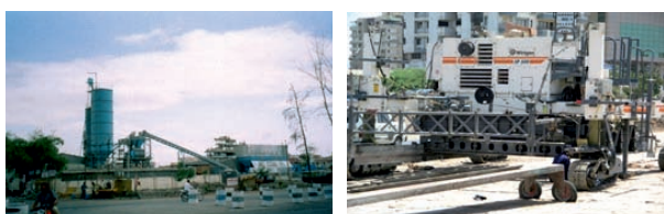
Figure 6: Batching Plant Of 120 Cu Mt/ Hr Capacity, 8 Mt Width Slipform Paver
