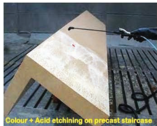
Figure 6: Colour + Acid etching on precast staircase
