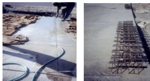
Figure 7: DLC Layer 150mm Thickness, Dowel Bar Caging, Dummy Groove Cutting
