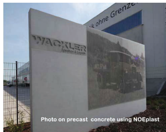
Figure 5: Photo on Precast Concrete using NOEplast
