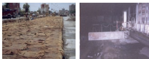
Figure 8: Curing with Jute Bags, Brooming and Curing Compound Sprinkling
