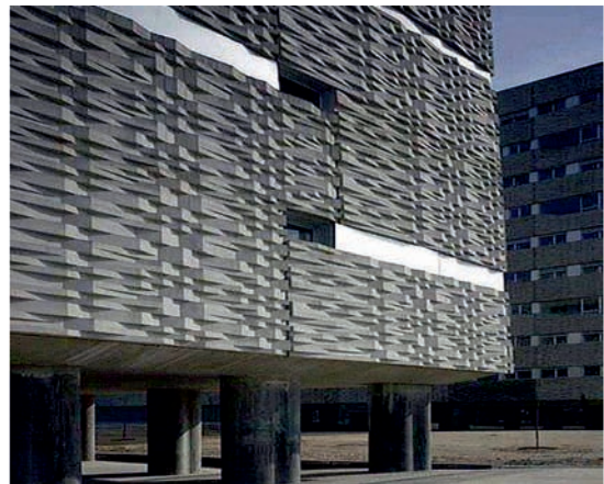
Figure 12: Architectural Concrete Outside Wall Faced
