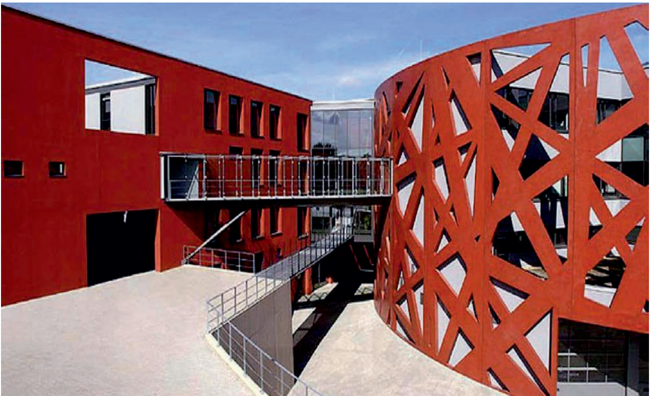
Figure 1: Architectural Precast for Cologne Fire Brigade Station
