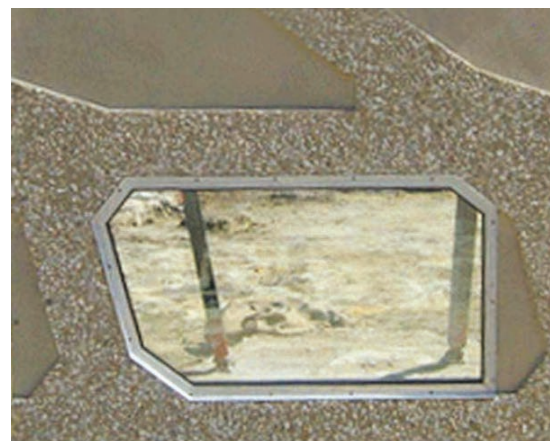
Figure 3: Colour (Pigment) + Design (Formliner)+Exposed Aggregate (Texture) on Precast Panel
