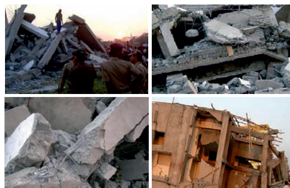
Figure 1: Failure of Structure Due to Earthquake
