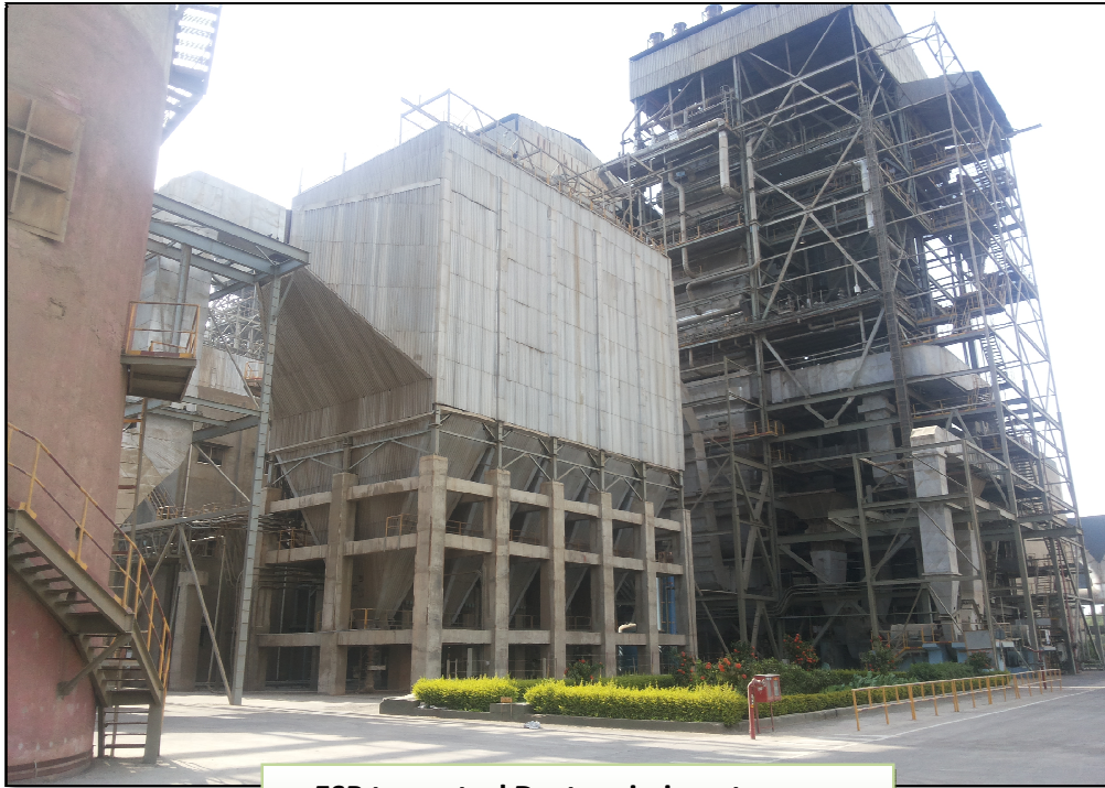
ESP to control Dust emission at source
